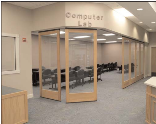
Hufcor GT Timberframed panels are used to create a private computer lab in this Florida library. The system includes an inline pass door and segmented panels that match the overhead soffit.
