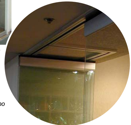
Glass panels are stored on a stack when not needed.
